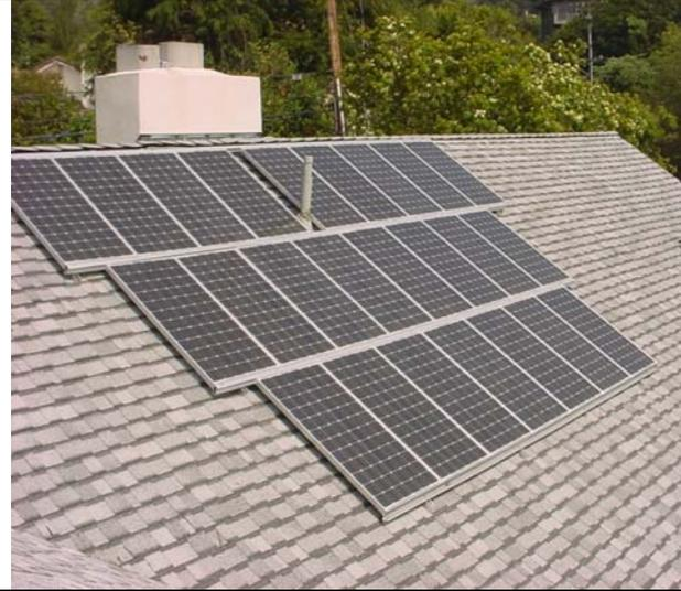
**A:** Modules may be racked in either portrait or landscape modes with the CompRail system. Ideally, the modules should be racked in portrait with their short edge in line with the axis of the CompRail™. This configuration minimizes the amount of rail needed to rack the modules and limits the number of feet and roof penetrations required.
