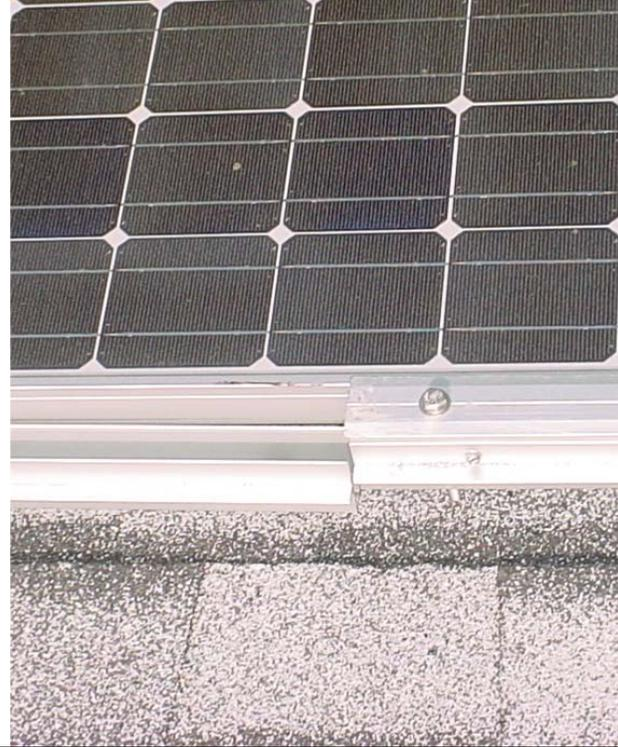
In instances where the row length exceeds the standard 264" length of the CompRail™, adjacent rails may be spliced together. With Comprail™ a separate splice connector kit is not required. Instead, the PV module frame is used to splice two rails together. The PV frame aligns and provides the support to hold the rails together until they are secured to the next strut foot/runner on the roof. A partially assembled splice is shown in the photo on the left.
