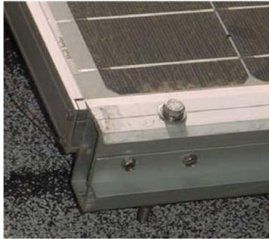
If the free edge rails (those with PV modules on only one side) were simply compressed, the upper rail would tend to bend over onto the free edge instead of clamping directly on the module. To prevent this, the free edge must be fixed with tek screws (self tapping sheet metal screws) or rivets.
