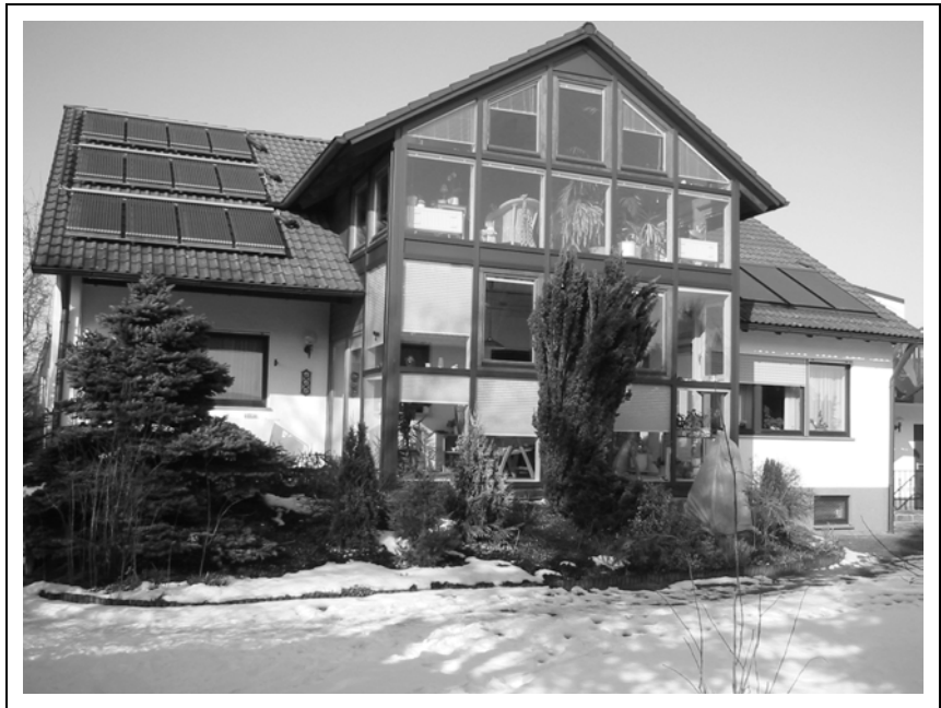
Figure 1 : Two-family House with Solar Installations
