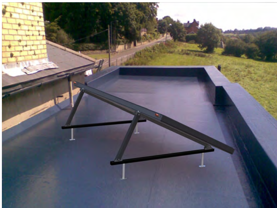
SunEarth Landscape Rack Flat Roof Installation
